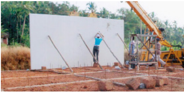
GFRG wall panels being placed with the help of cranes
